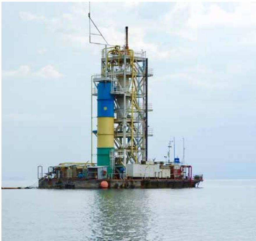
Methane extraction platform at Lake Kivu
