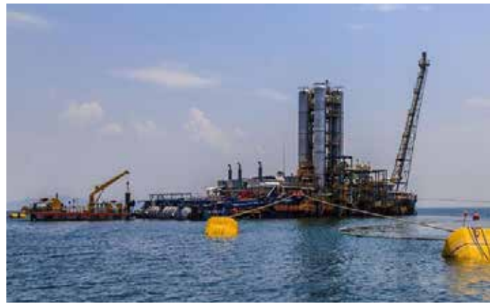
Methane Gas extraction Plant
