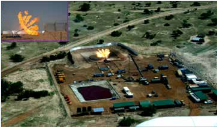
Figure 7: Drill Stem Testing at Kasamene (right) and well log section (left).
