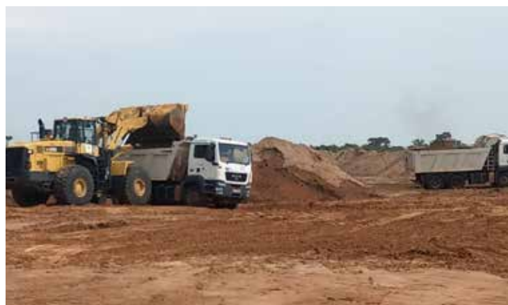
Central Processing Facility construction in Tilenga Project
