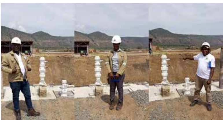
Pad 2 construction in Kingfisher Development Area
